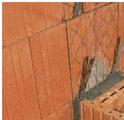
Wall connection: butt joint with flat steel core and fully grouted butt joint or even better: slot connection in the outer wall
