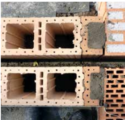
Chambers of non-full size (eg in the case of passages at the ends of walls or in the masonry verge) are to be crammed in layers with masonry mortar MG III or MG IIa in layers.
