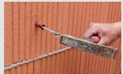
Hammer in dowels flush with hammer.
