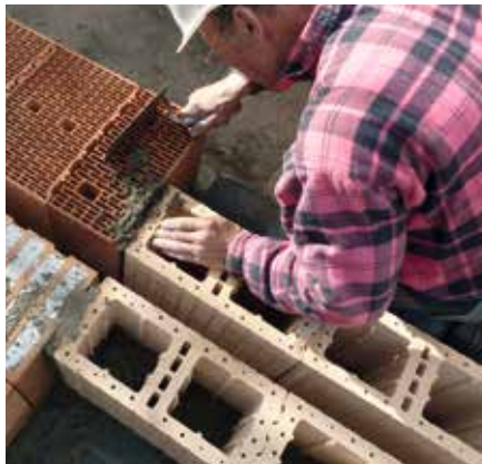
For wall connections by means of butt joint (Example, two-shell house partition), the connecting joints are full to mortify (joint thickness about 1.5 to 2.0 cm).
