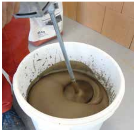
The thin bed mortar is ideally mixed with a powerful stirrer and double stirrer with no lumps.
