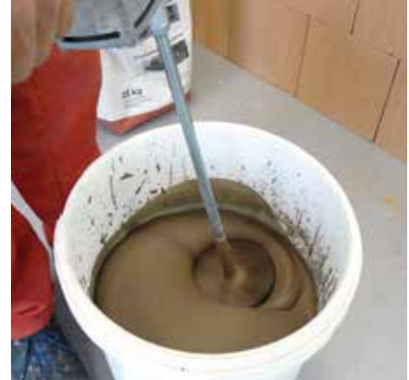
If possible, mix the Poroton thin-board mortar in a sack bucket with a powerful mixer.
