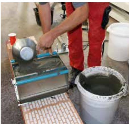
The stirred thin bed mortar is filled into the mortar roll. Before starting work, spray the mortar roll with release agent! Facilitates the later cleaning.
