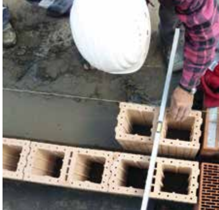
Leveling and leveling of the 1st tile layer on the leveling mortar layer (example bivalve house partition wall).
