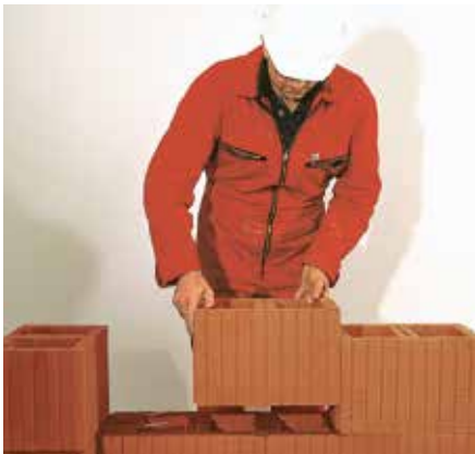
Dip the PFZ-T into the thin board mortar with the underside and move. The mortar must adhere fully to the webs. Alternatively, the mortar can be applied with a roller on the bearing surfaces of the brick.
