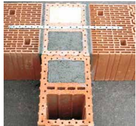
The most economically sound connection of single-shell apartment partitions to monolithic exterior walls is the integration with thermally insulated beginners (details see next page).
