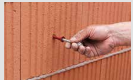
Place dowel (if necessary already with screw).
