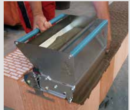
Rolls: Simple and efficient application of the covering thin-bed mortar
