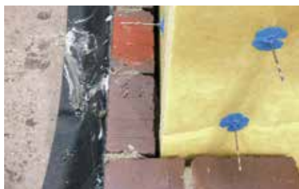
Picture 5 Clamping disc with drip-off nose as insulation attachment
