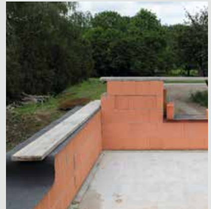
Window parapets and masonry crowns are to be protected during the construction phase against the ingress of the day water (rain and snow).
