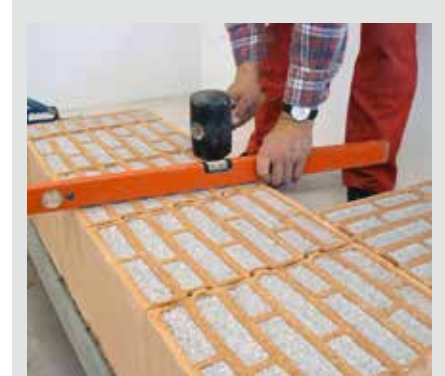
The 1st layer: Align horizontally in the mortar bed
