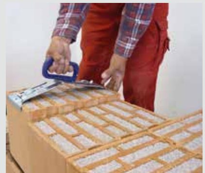
Setting: Simply place bricks in the teeth of the neighboring tile Carrying aids: make placing more comfortable
