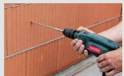
Drilling without impact function with sharpened carbide drill.
