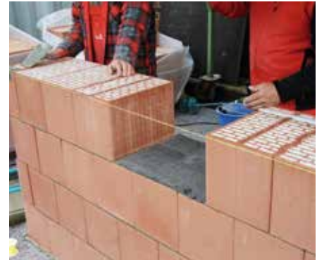
Bituminous roofing membrane R500 in thin-bed mortar laid on Poroton-T7-P
