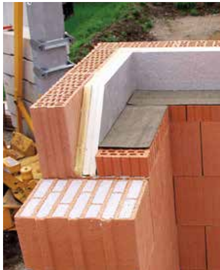
Ceiling support with ceiling bricks
