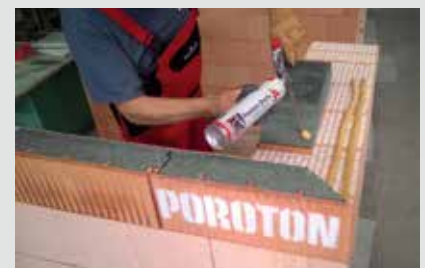
To stabilize the corner area, glue the cut surface to Poroton Dryfix Glue.
