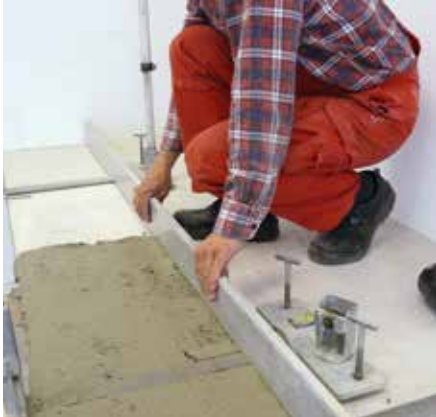
Apply the leveling mortar layer using Justierboy with normal mortar MG III.
