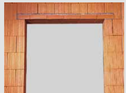
Walling, clay flat lintel
