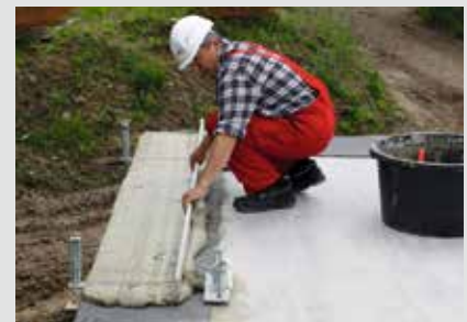
Justierboy: simplified and precise application of the 1st layer
