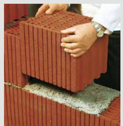
Laying the block
