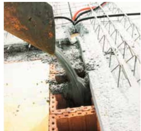
Finally, fill the created wall with concrete in a single operation. This is done efficiently when concreting the ceiling structures.
